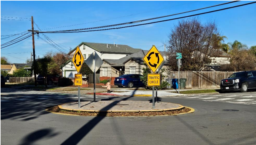
Example of a Traffic Circle – City of Hollister. Photo by Kimley-Horn
